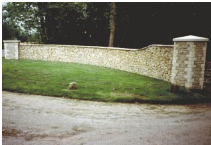
Walling at Salperton Park Estate
